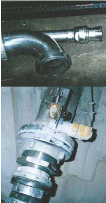
Unloading nozzle hose attached to silo feeder pipe using an adapter between the hose and the pipe.
